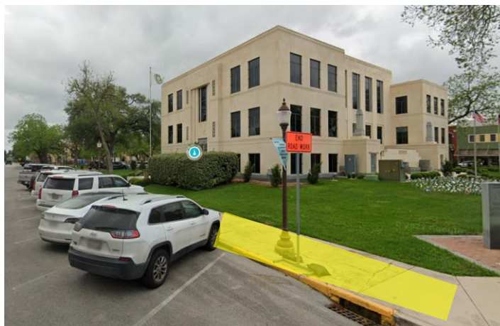
Guadalupe County Courthouse at 101 E. Court Street, Seguin, TX
